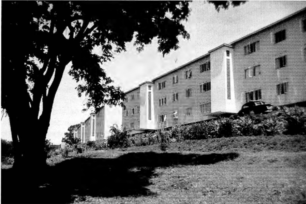
Figure 15.6 May's Delamere Flats Apartment Buildings, Nairobi, designed 1938–39, built 1947–51
