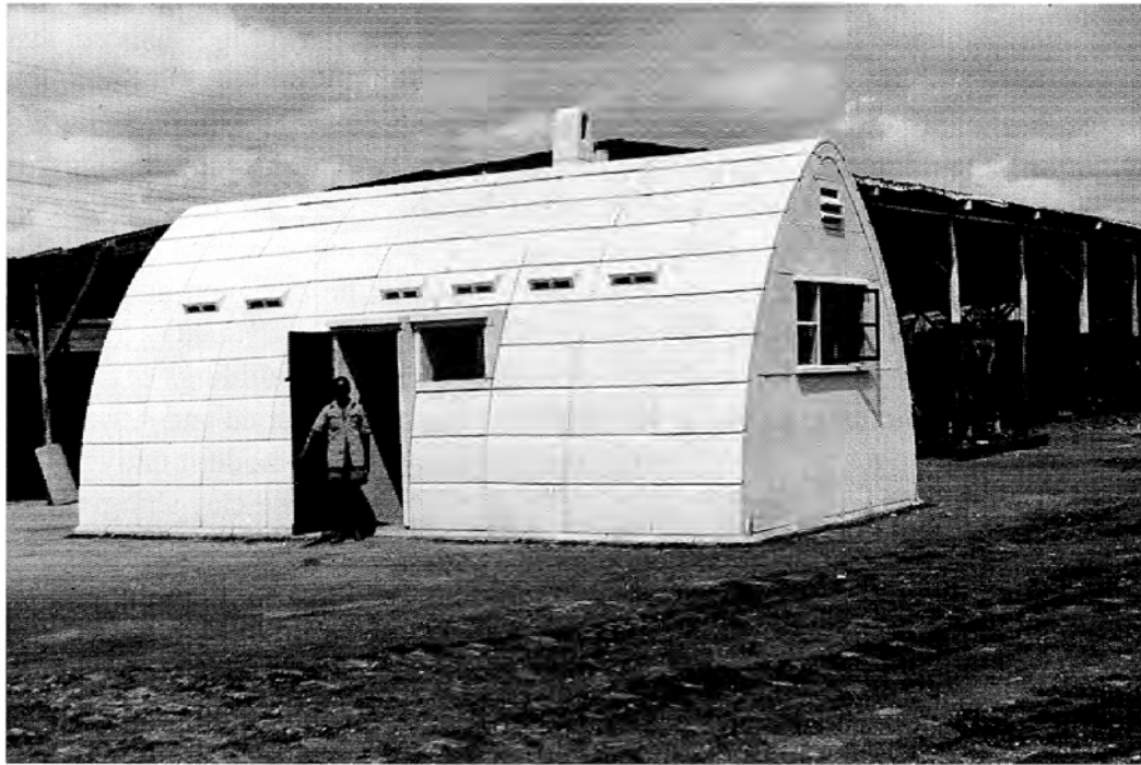
Figure 15.10 May's "Hook-on-Slab" concrete-panel huts for Africans, 1945
